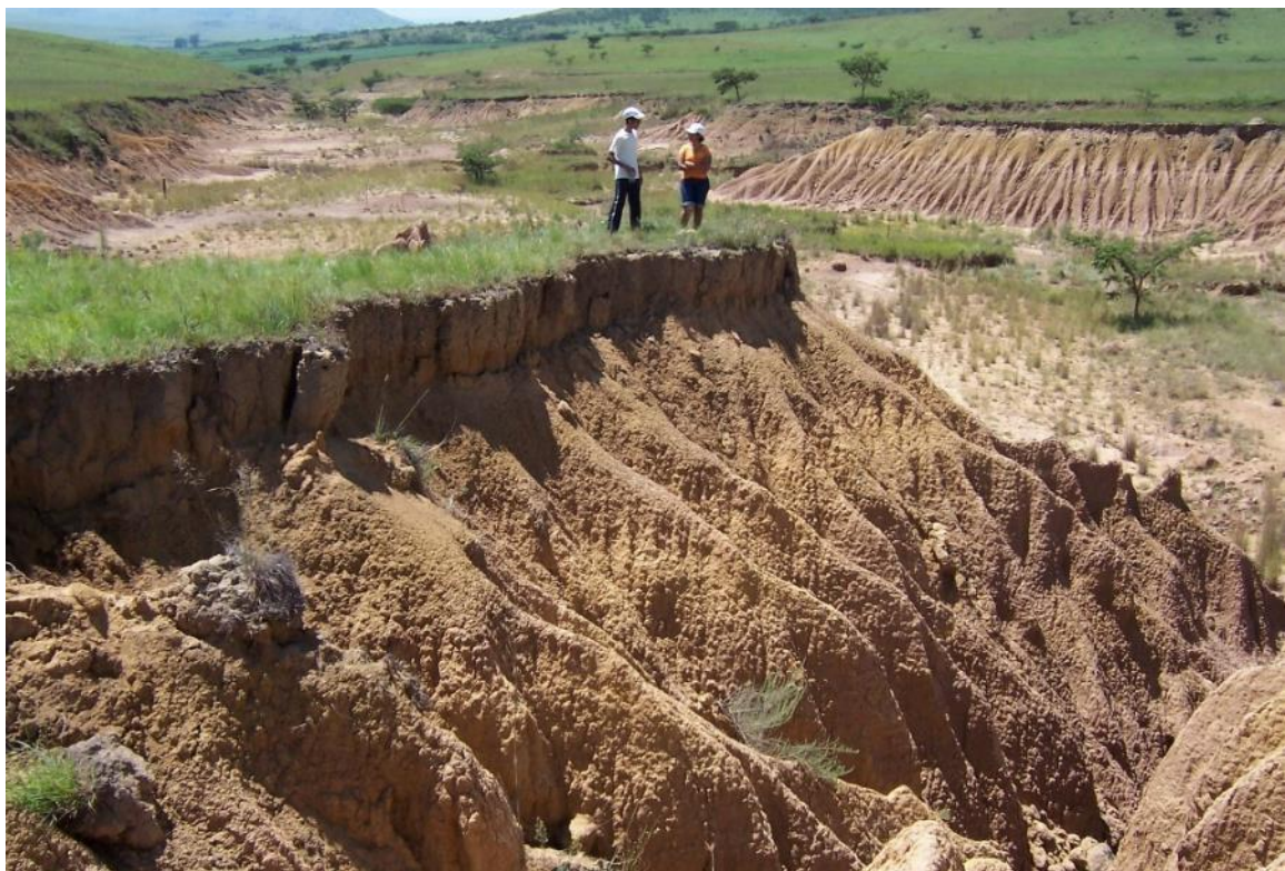
Figure 2.7. Severe gully erosion near Mabhulesini in the Upper Thukela Catchment (Photo: Joshua Weiss).
